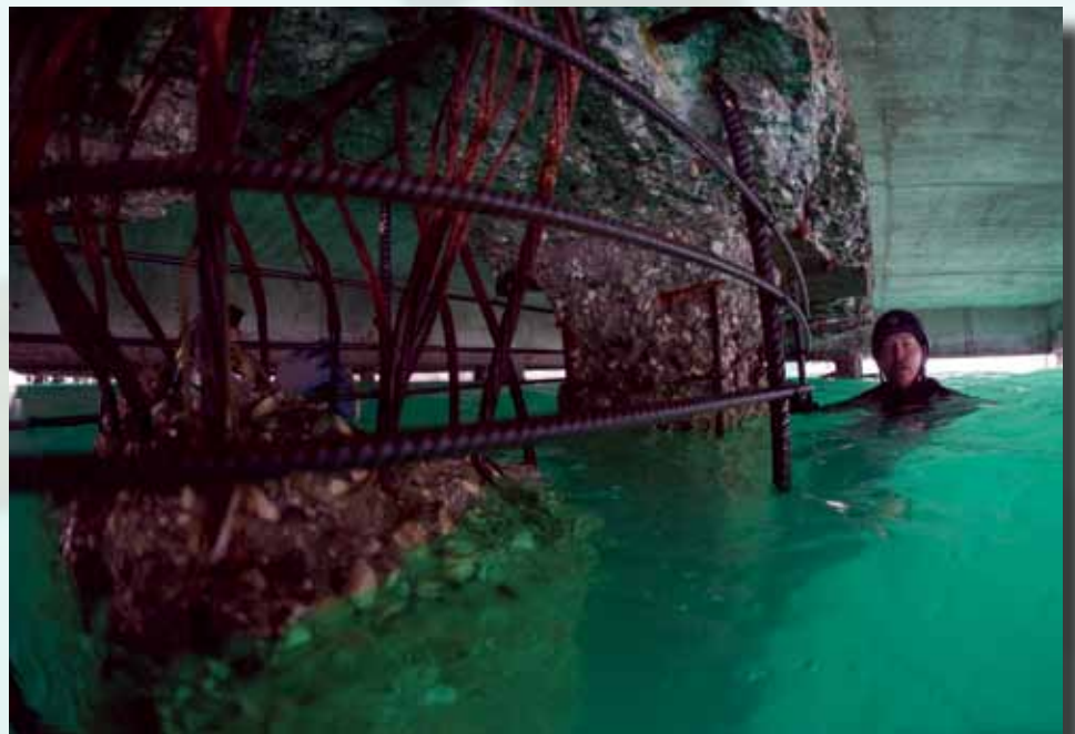
EOC(SCW/DV) Hurley & EOC(SCW/DV) Eckroth performing quality control inspections of pile-cap, repair, and formwork. Photo by MC2 Christopher Lussier NECC Det Combat Camera Norfolk, Dive Locker.
