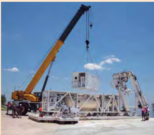
SAT FADS main Deck Decompression Chamber being assembled on pier next to Naval Experimental Diving Unit.
