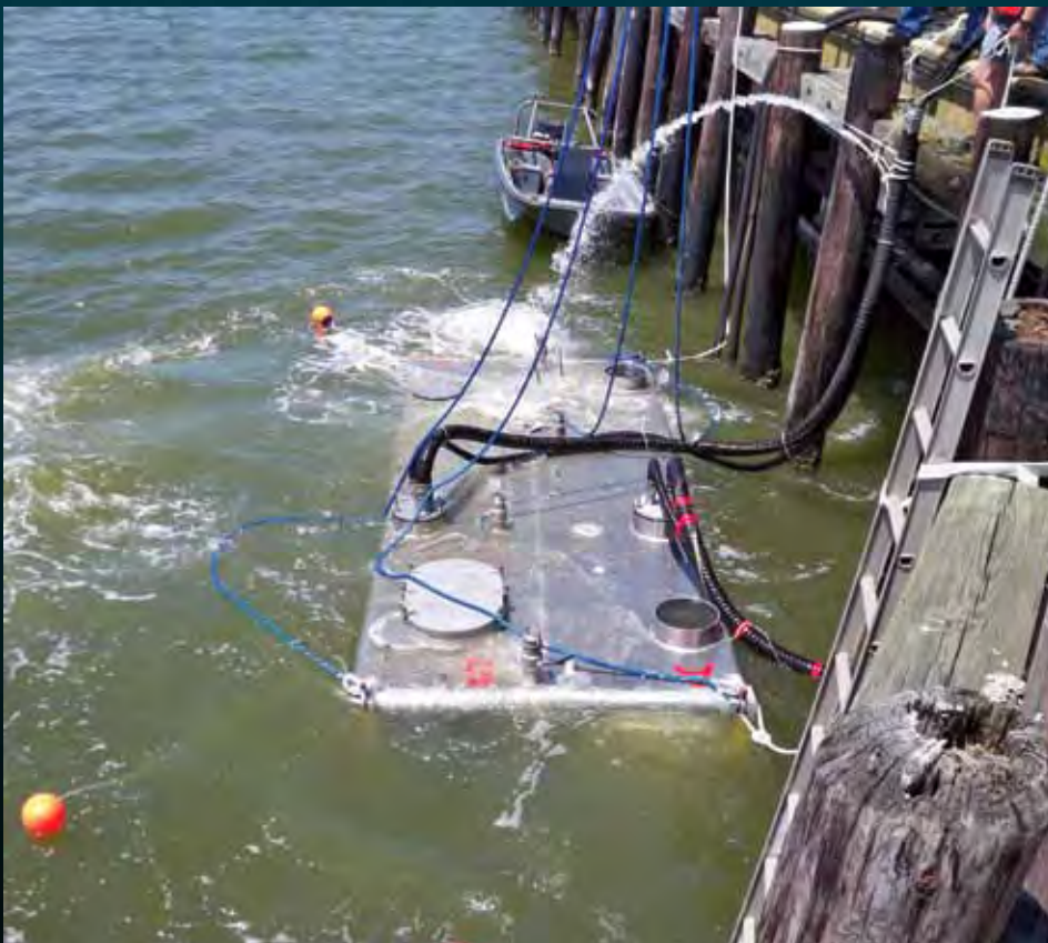
New salvage project affectionately nicknamed the 'Hulk' rigged for salvage operations.
