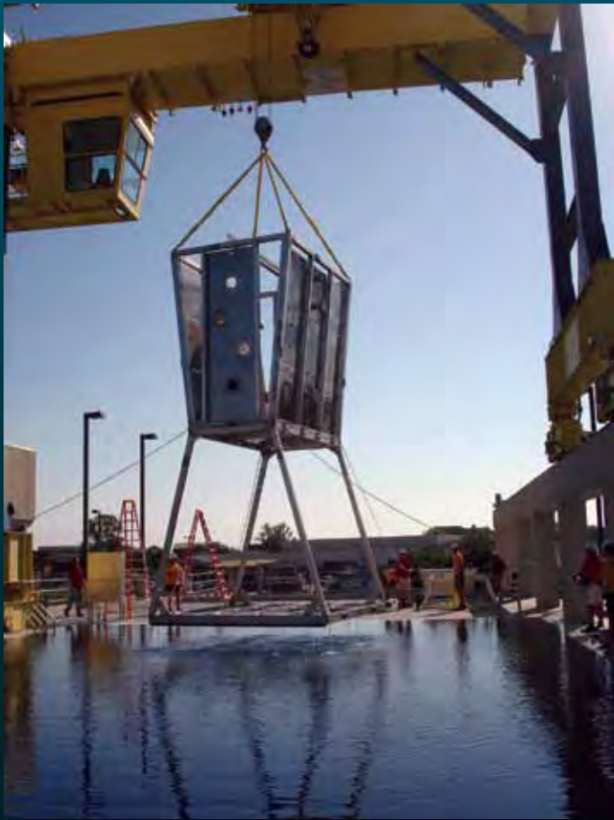
Ship Husbandry project rigged with lower module stand attached into the new pool.
