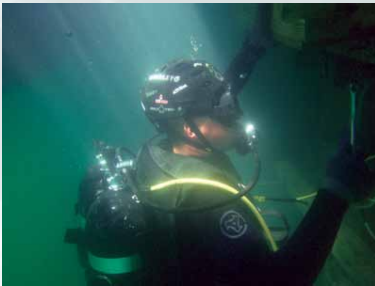
PFC Winters, U.S. Army, secures friction clamps to support concrete form work weighing several thousand pounds. Photo by CE3(SCW/DV) Dailey.
