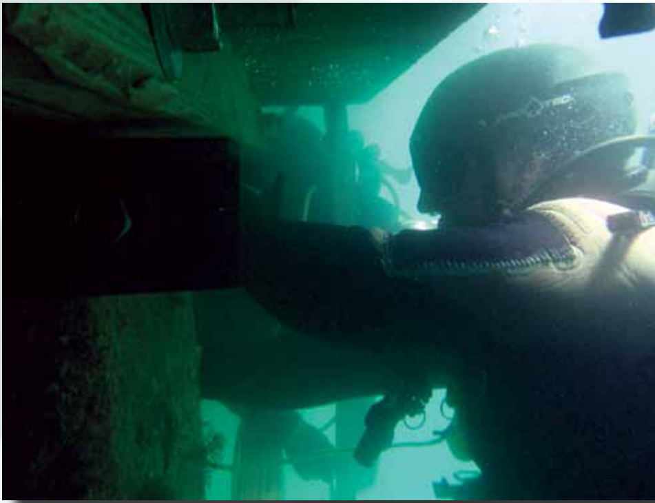
EA2(SCW/DV) Robins secures friction clamps that support concrete forms weighing several thousand pounds. Photo by CE3(SCW/DV) Dailey.
